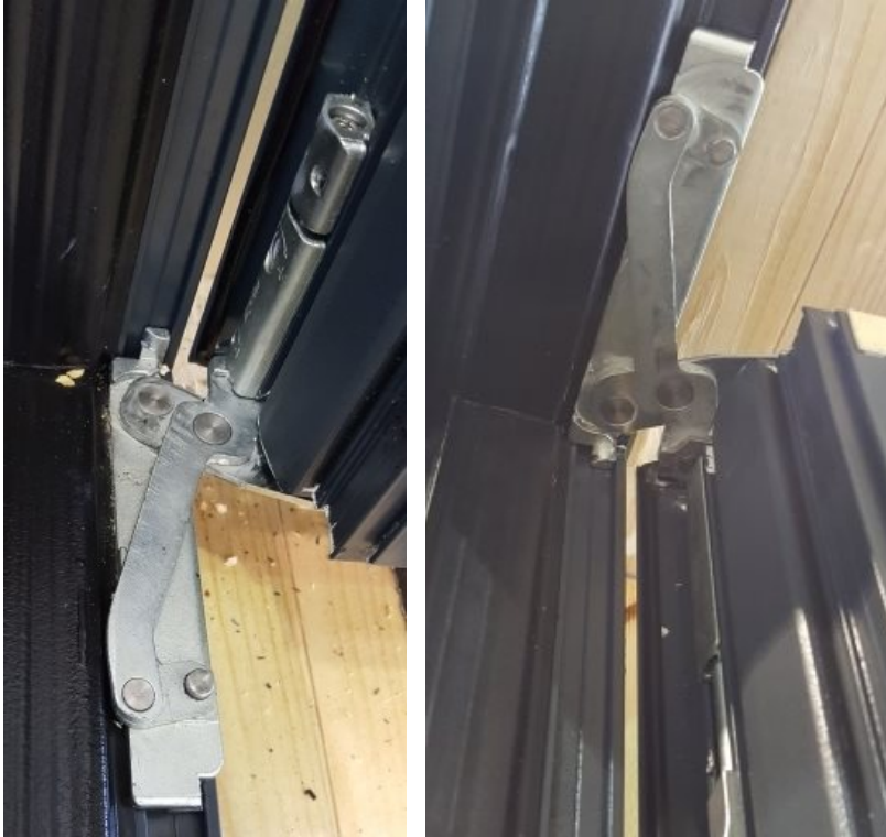
Hinges – Left, Bottom Hinge; Right, Top Hinge
