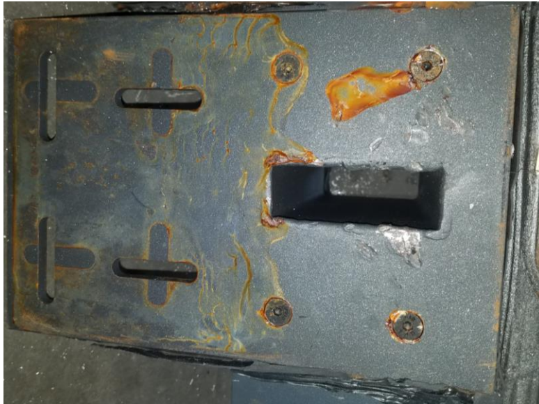
Installation plate for mullion
