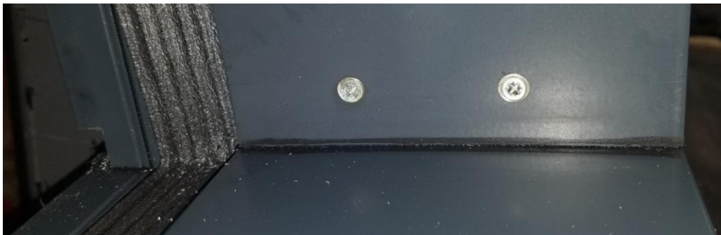
Screws for the horizontal mullion in to shear block
