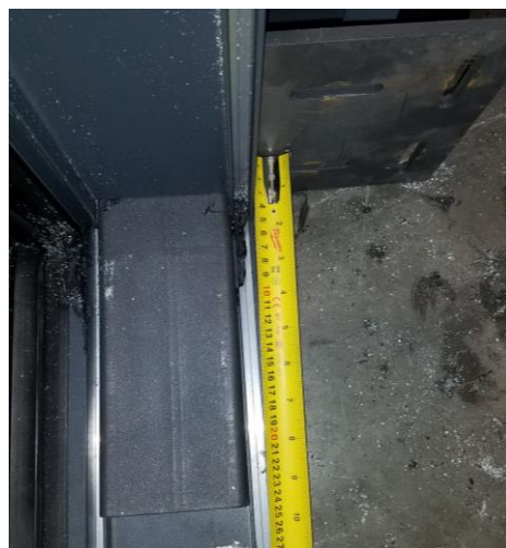
Steel rectangular profile welded to install plate, inserted into the jamb
