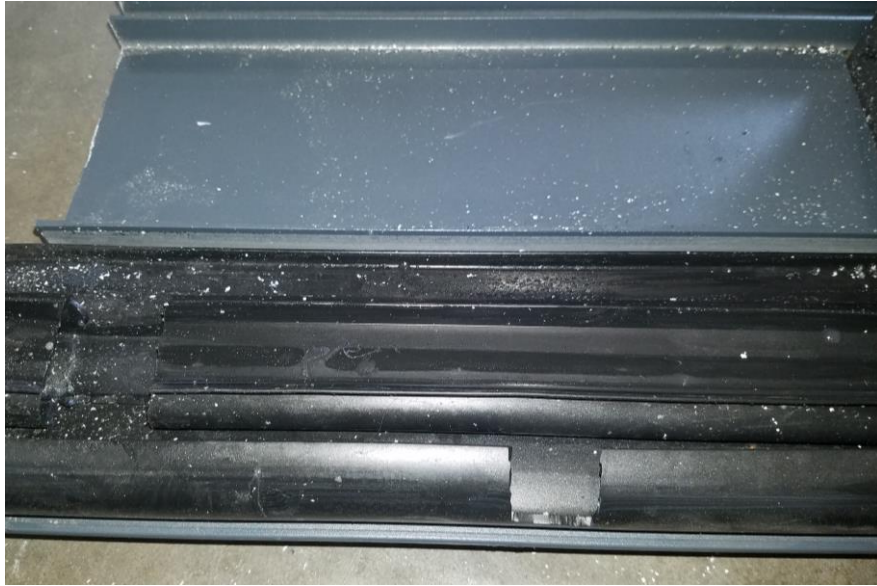
Drain slots cut into sill gaskets
