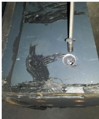
Installation plate secured to the jambs
