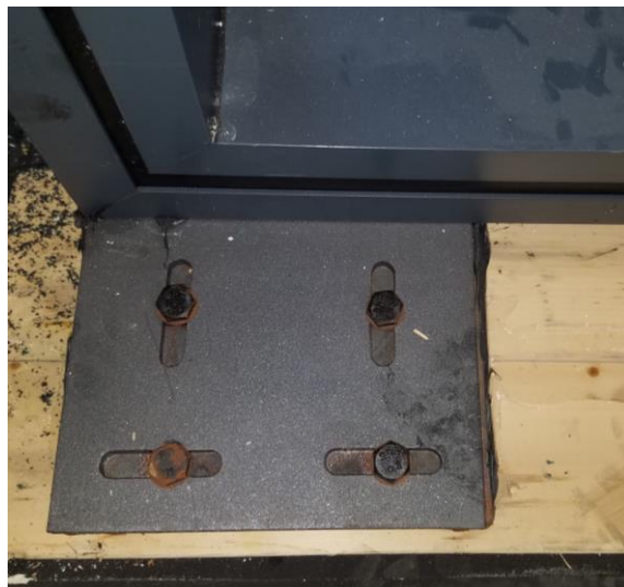
Installation plate bolted to the steel buck
