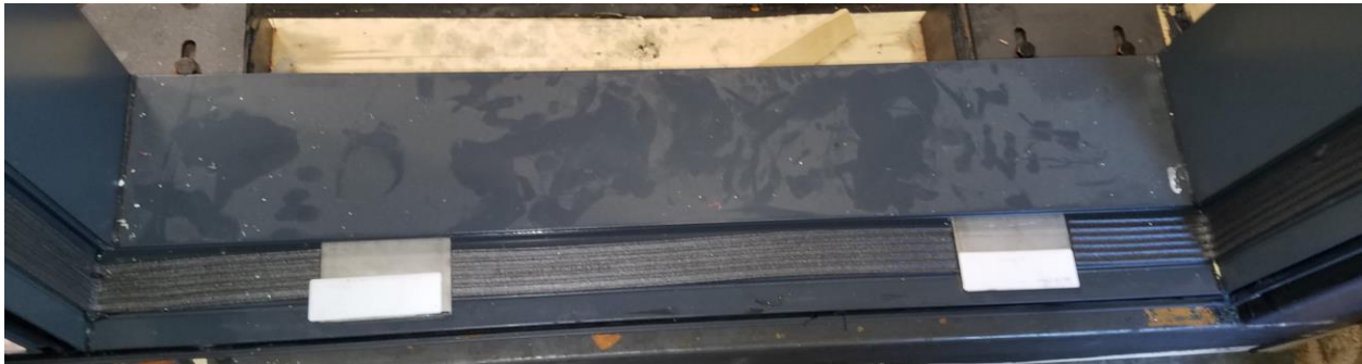
Setting blocks on aluminum carriers
