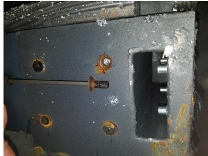
Installation plate secured to the sill
