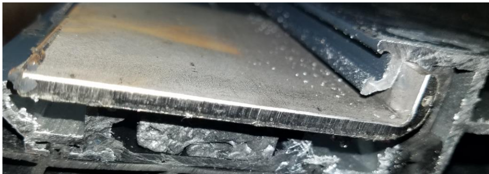
Aluminum setting block carrier
